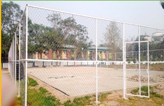
New Basketball Court under construction at KV AFS Digaru
